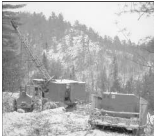
Drilling continues at URSA Major's Shakespeare project.
